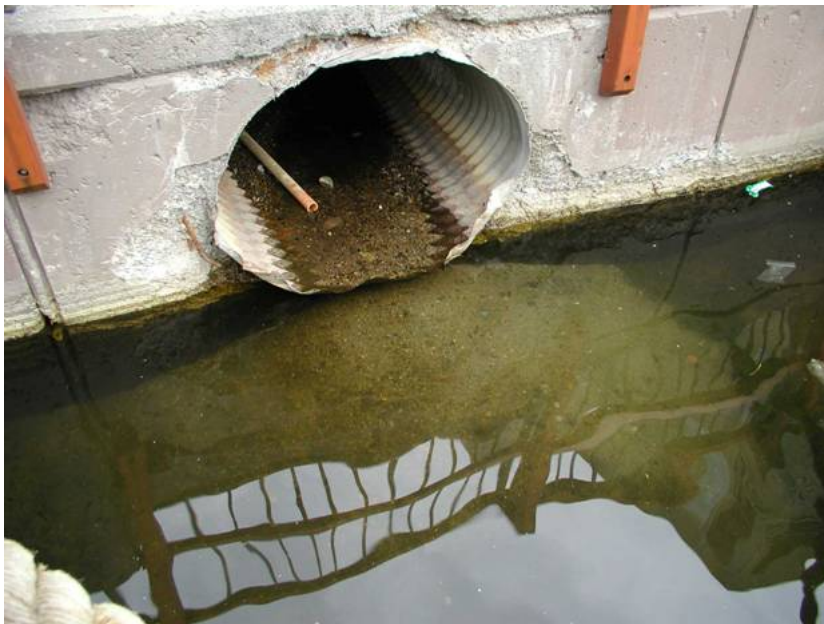
Figure 5. Bedload sediment accumulation in sewerage and near inlet to pond (Snowmass, CO).
